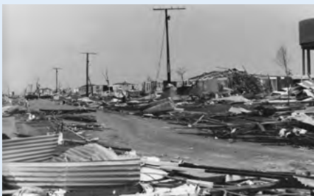
A Darwin suburban street after a grader had been through the street. (Public domain)
