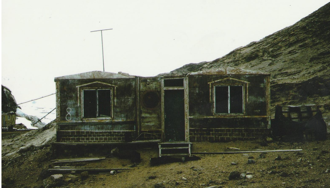
Russia – ПРОГРЕССЙ “Progress” 2 Station – “Old Station”
